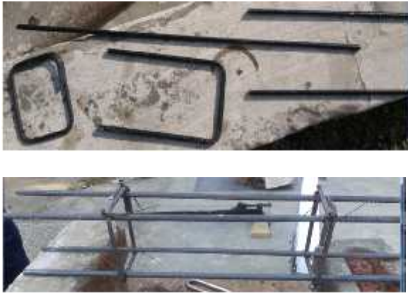
Figure 3.47 Edge beam reinforcement and beam cage
