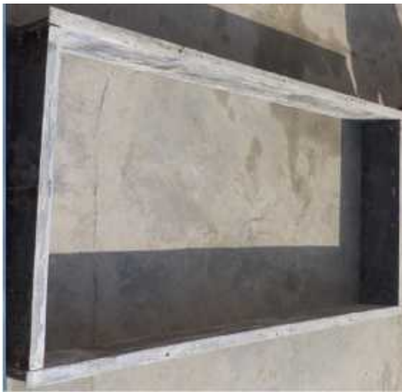
Figure 3.45 Finished form for casting
