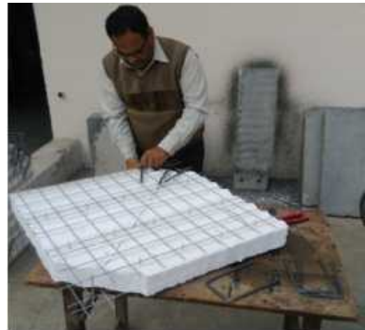
Figure 3.9 Measurement for cutting EPS panel to the required size and shape
