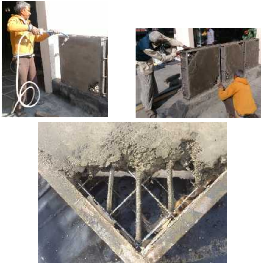
Figure 3.18 Cleaning of corners using air-blast before filling
