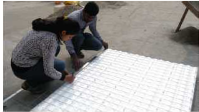
Figure 3.9 Measurement for cutting EPS panel to the required size and shape
