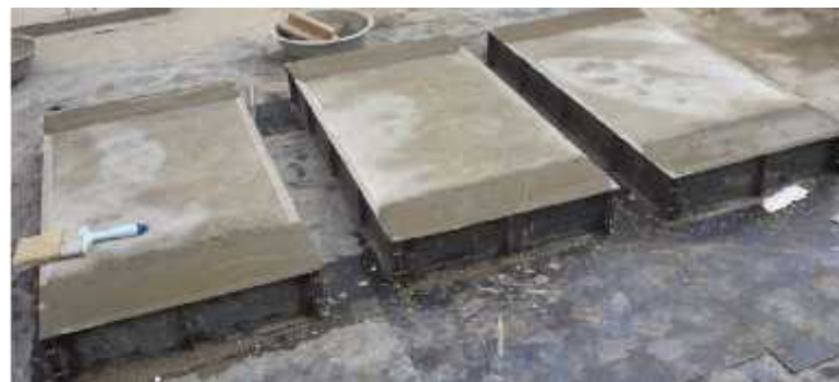
Figure 3.50 Casting of edge beam
