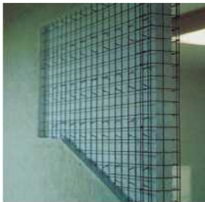
Figure-1.4 Wall panel
