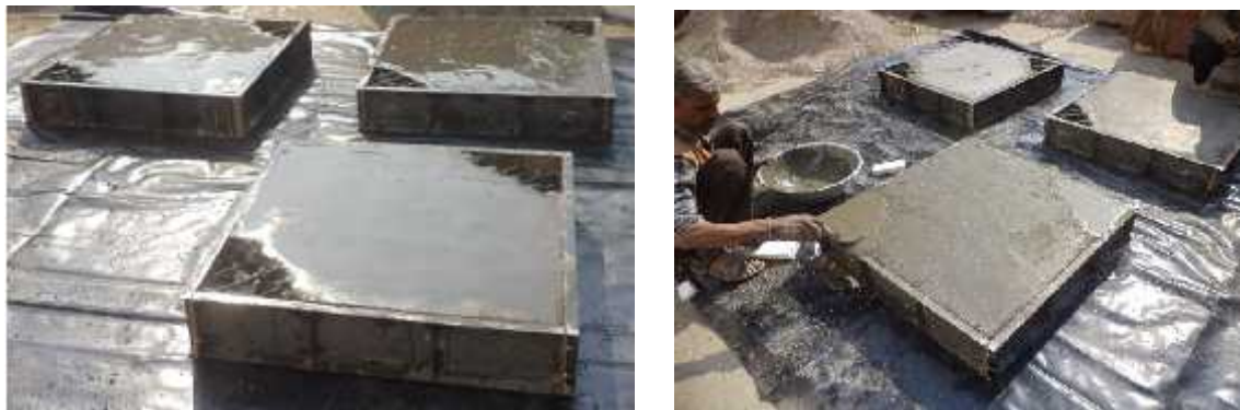
Figure 3.19 Filling of corners
