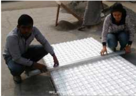
Figure 3.9 Measurement for cutting EPS panel to the required size and shape
